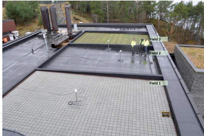
Figure 15. KLIMA 2050 project field test at Høvringen using LECA® LWA in Trondheim, Norway (field 1—LECA® LWA below permeable paving blocks; field 2—Black empty reference roof; field 3—LECA® LWA under a traditional sedum green roof) (Photo: Tore Kvande, NTNU—Norwegian University of Science and Technology).
