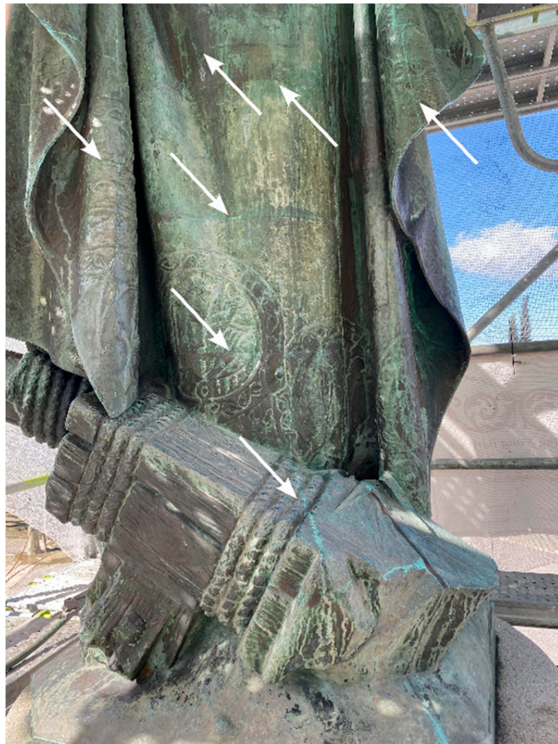
Figure 2. Detail of the sculpture showing the separation lines (identified by arrows) between the different sections.
